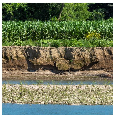
Eroding river banks near Fillmore, NY.
