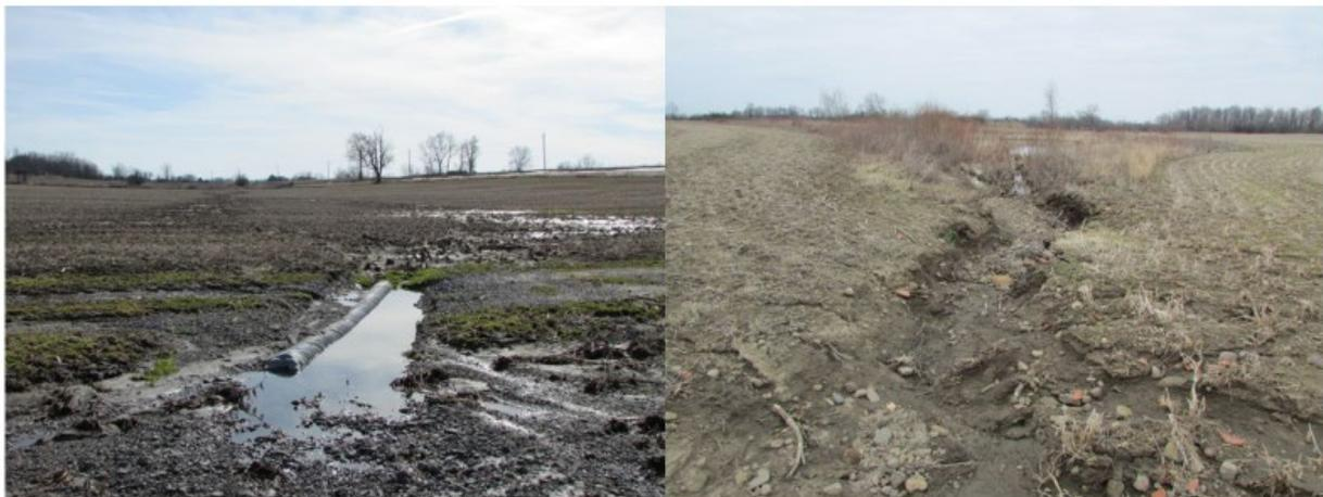
**Figure 1:** These pictures show the erosion at the site of the first project. This 85 acre field is currently being excavated to install grassed waterways, WASCOBs, and underground outlets.
